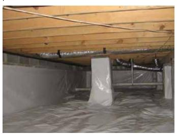
NOTE: Completely sealed crawl spaces (no exterior crossventilation) require a dehumidification system as part of the sealed crawl space design.
