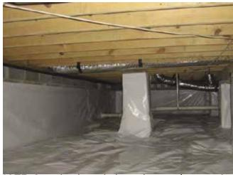
NOTE: Completely sealed crawlspaces (no exterior cross-ventilation) require a dehumidification system as part of the sealed crawlspace design.
